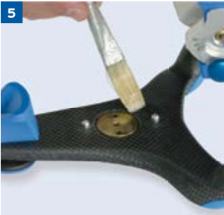
5 Insulate the carbon surface in the area of the adhesive plate by applying a thin layer of petroleum jelly
